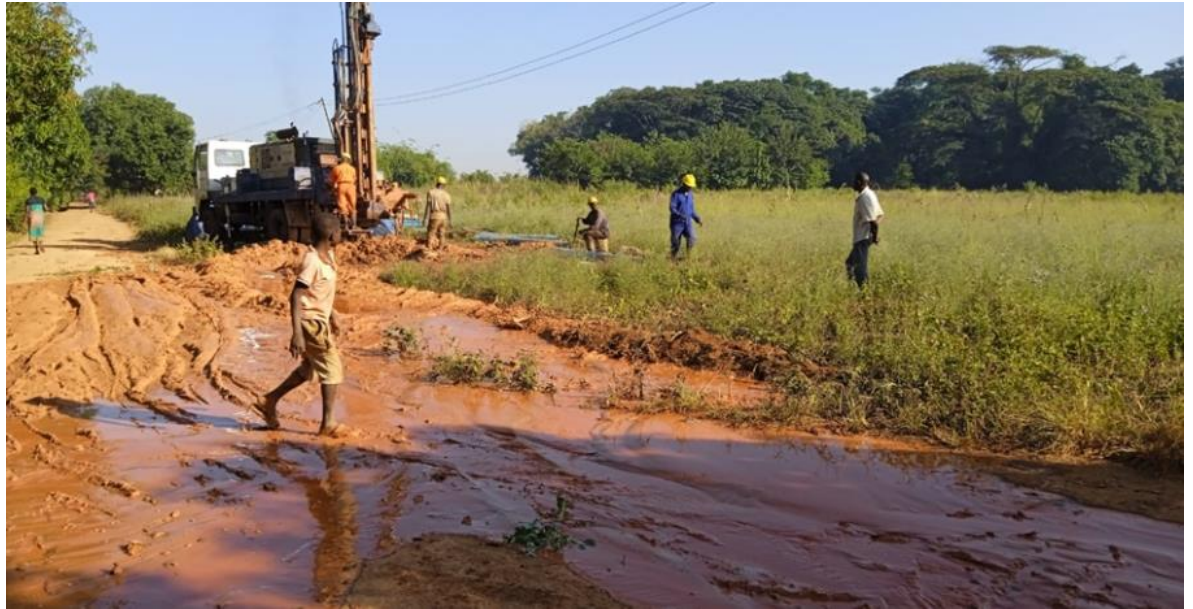
A borehole being drilled
