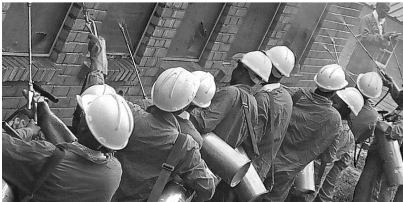
Employed spray operators are being trained on spraying technics, human and environmental safety and documentation of data collection tools.
